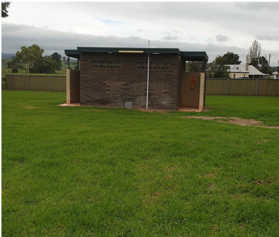
Photograph 2 - Old brick toilet block in McMasters Park
