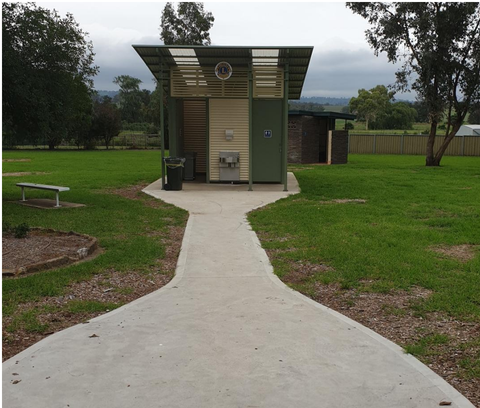
Photograph 1 – New toilet block in McMasters Park erected by the Coolah Lions Club
